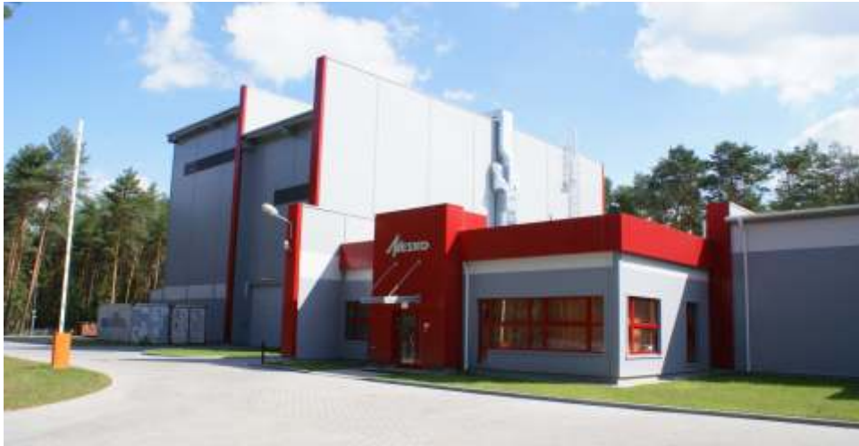
The demilitarization plant for useless fighting materials
